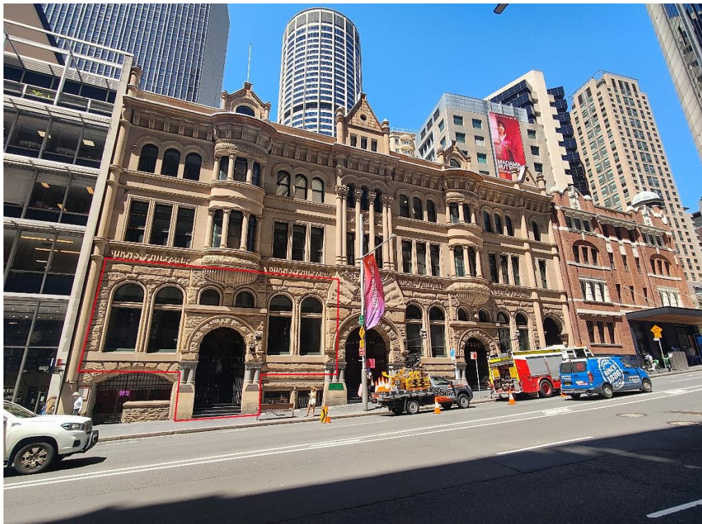
Figure 2: The site viewed from Bridge Street. The approximate extent of the subject tenancy is outlined in red.
