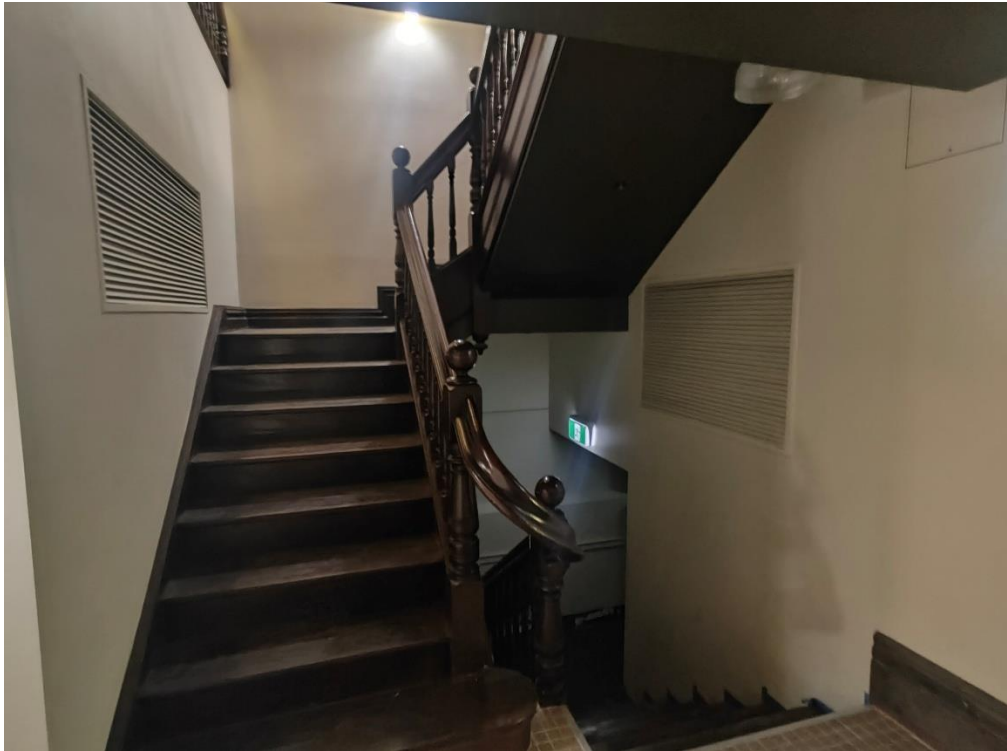
Figure 7: The existing staircase to be retained connecting the ground and mezzanine levels
